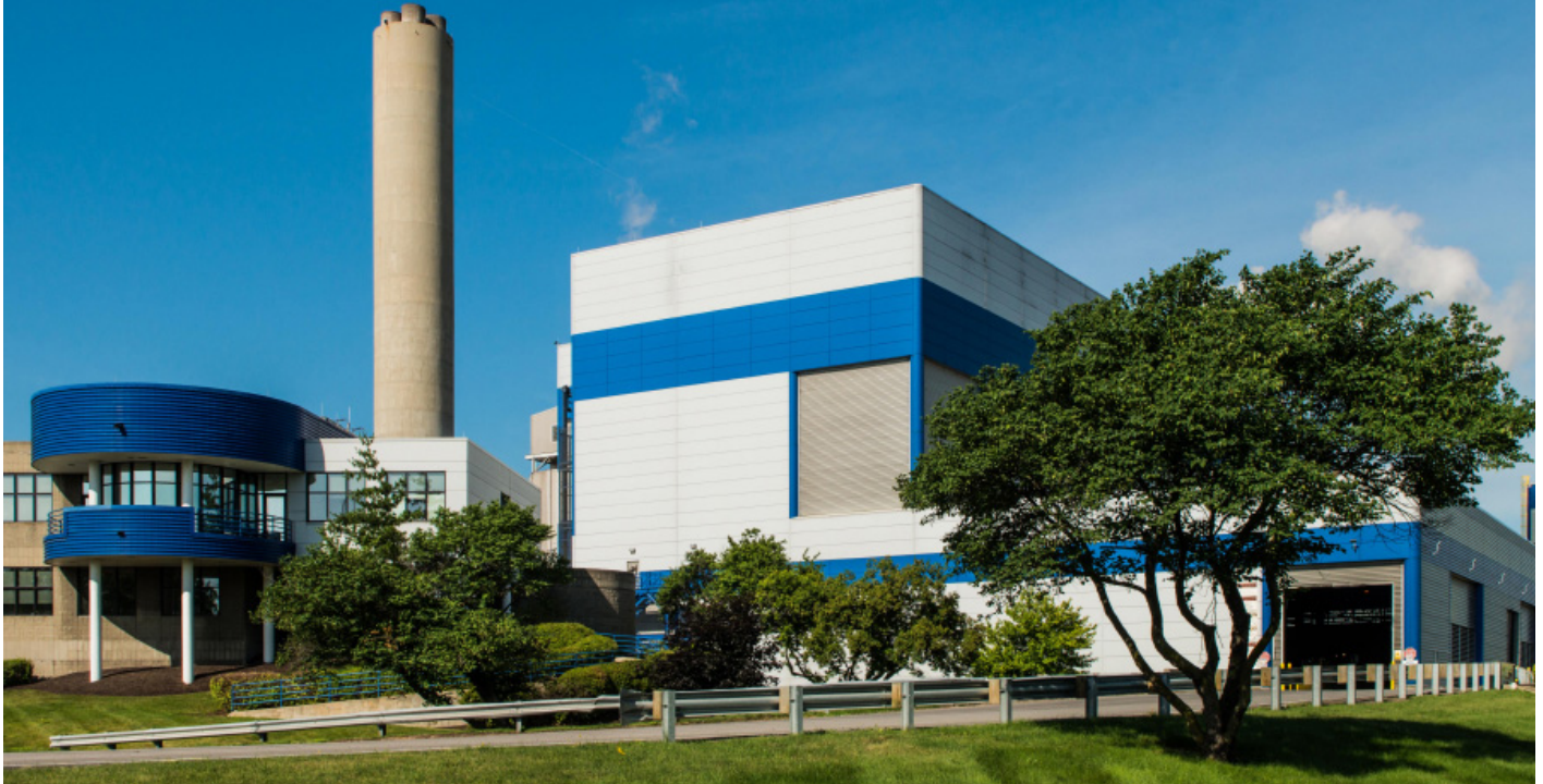
Covanta Indianapolis EfW facility
