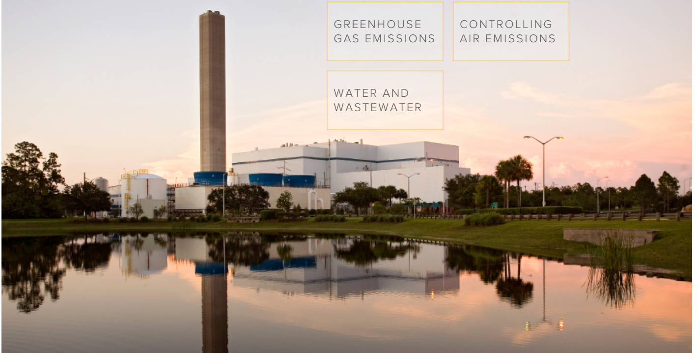
Lee County Solid Waste Resource Recovery Facility
